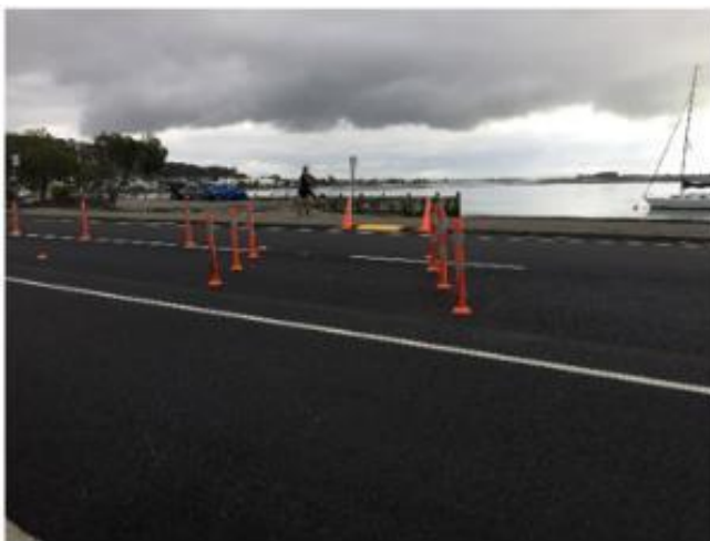
Pedestrian refuge using reflective bollards
